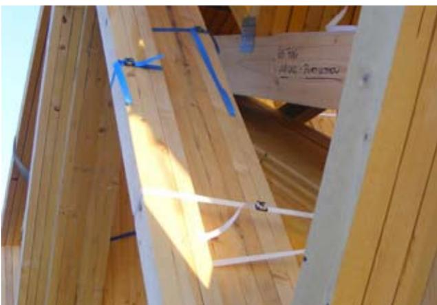
Figure 1 Colour-coded-banding system
